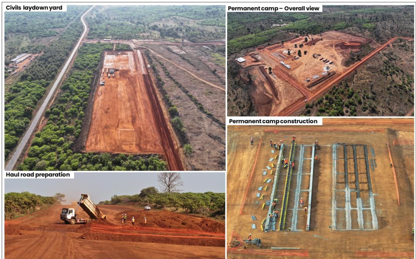
Figure 2: Early works underway
