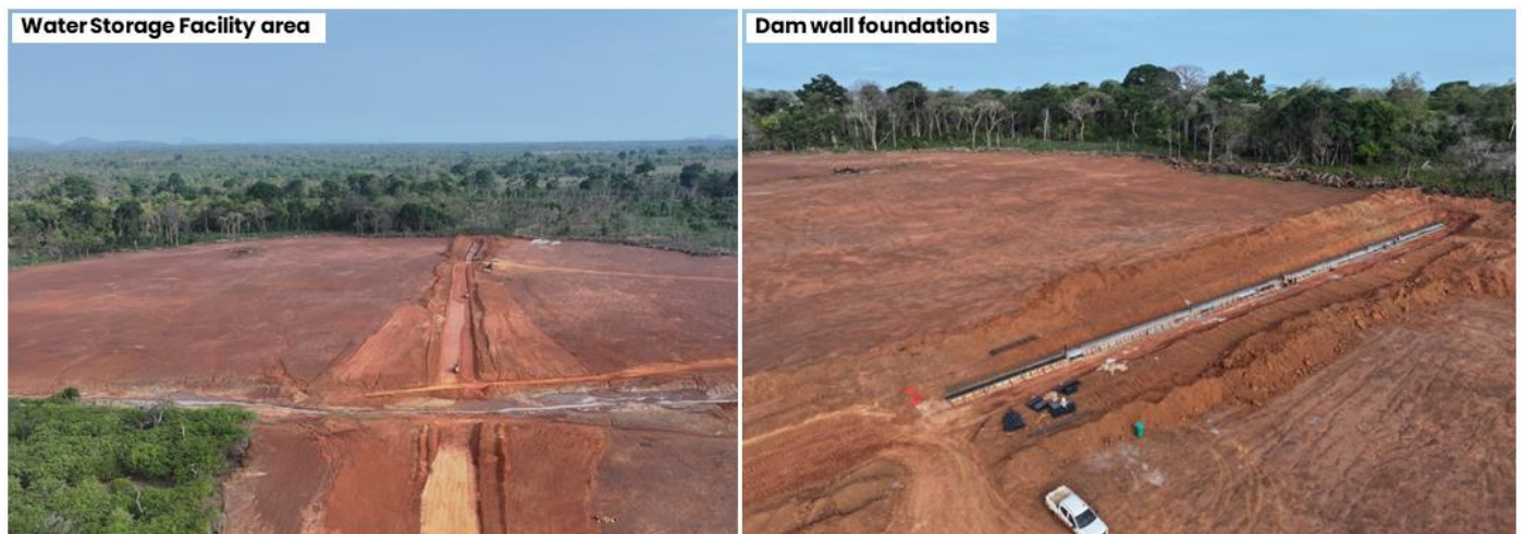
Figure 4: Water Storage Facility preparation
