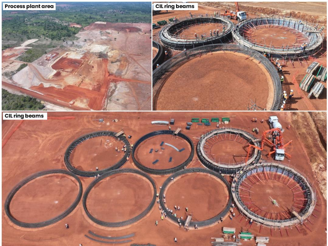
Figure 1: Process plant area overview and CIL ring beams
