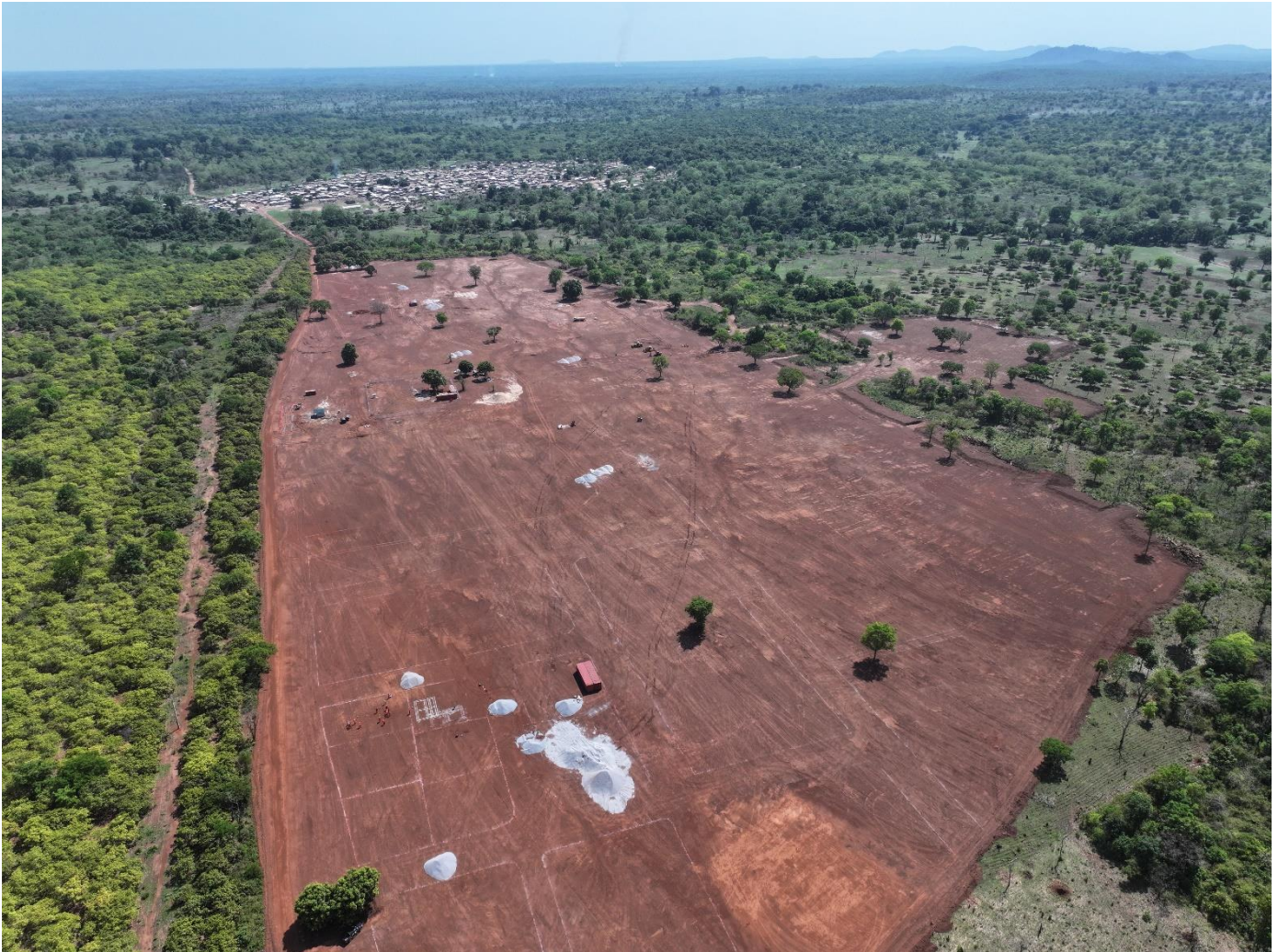
Figure 7: Resettlement area preparation and early works
