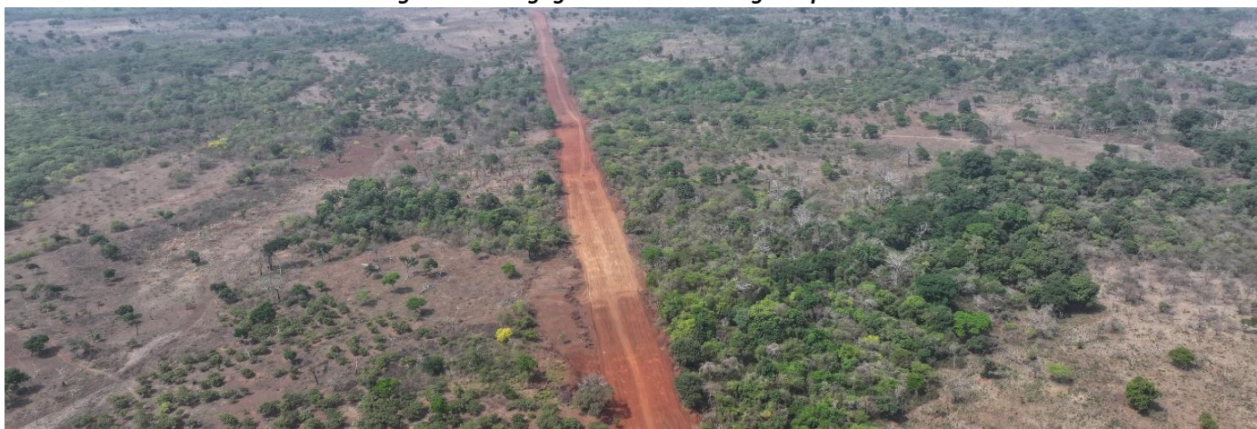
Figure 6: Gbongogo haul road nearing completion
