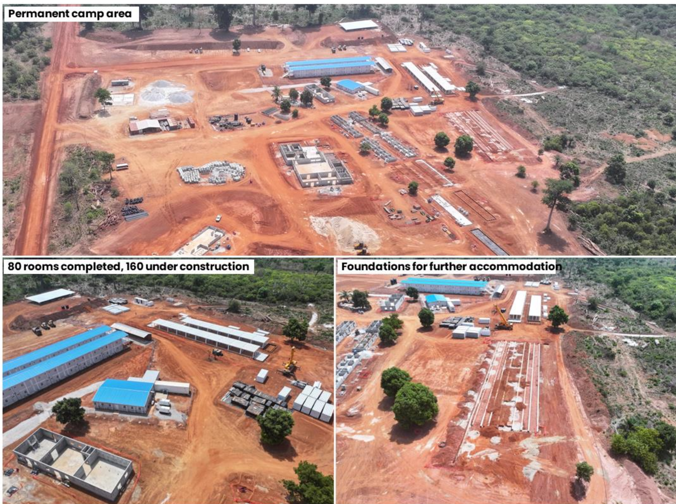
Figure 5: Permanent camp construction progress
